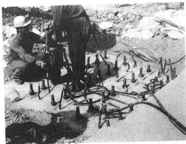
Fig 7 Abutment vertical prestressing (Bars \phi 50 mm.)
