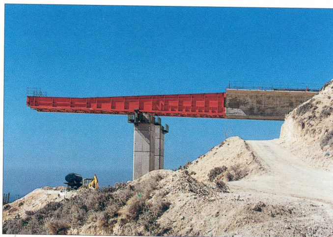
Fig. 5: Steel launching nose
