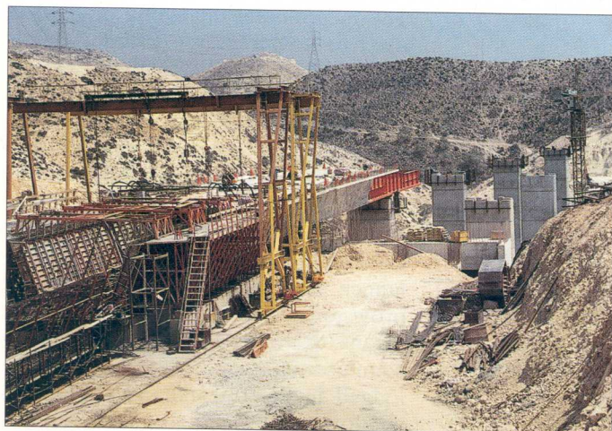
Fig. 4: General view of the casting yard
