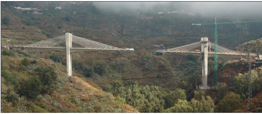
Fig. 5: Deck construction with the balanced cantilever system
