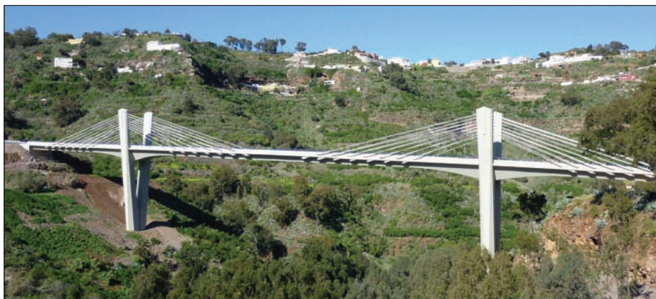
Fig. 1: General view of the Teror Viaduct
